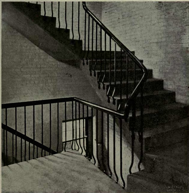
FIG. 175. — Concrete Stairs, Walter Baker Co.'s Building, Boston.
